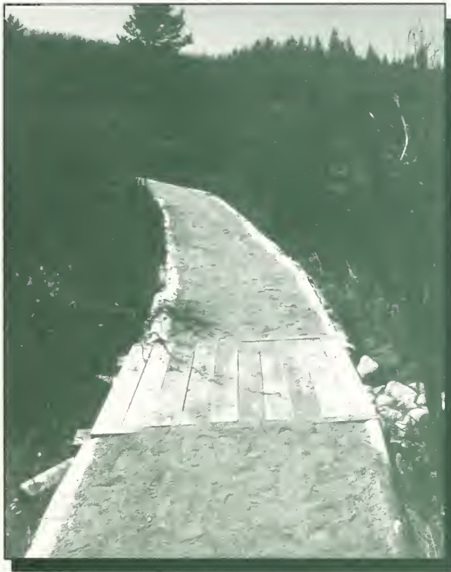
Figure 17—A new turnpike will need additional fill as it settles, especially during the first year. This turnpike has a timber culvert.
